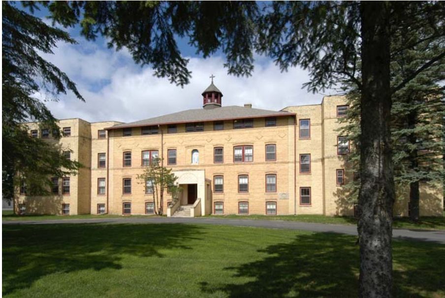
Figure 4: Restored main facade of Riverwood Pines Apartments. Photo from Preservation Alliance of Minnesota File Photo.
