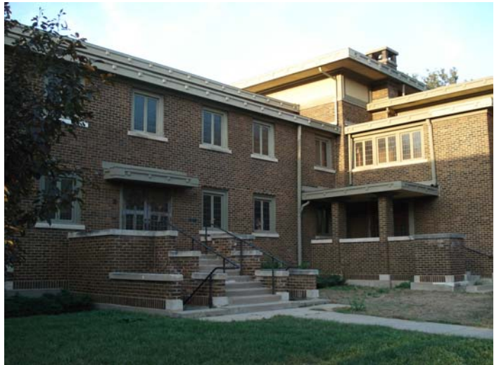
Figure 2: Restored Education Wing and Church. Photo by Emily Thomas
