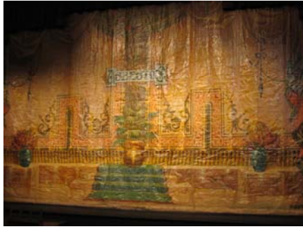
Figure 4: Encapsulated asbestos fire curtain. Photo by Author
