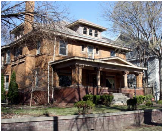
Samuel J. Hewson House Minneapolis
