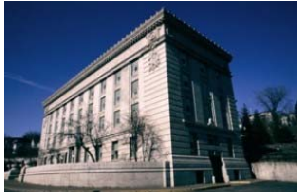
St. Louis County Jail Building Duluth
