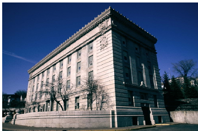
St. Louis County Jail, Duluth Vacant for 18 years, the County-owned Jail was headed for demolition. It has now been purchased by a private developer using the HRTC for commercial mixed-use putting it on the tax rolls for the first time in its history.
